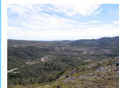
View from above the Mt William Reservoir along the route of the Stockton Tunnel
